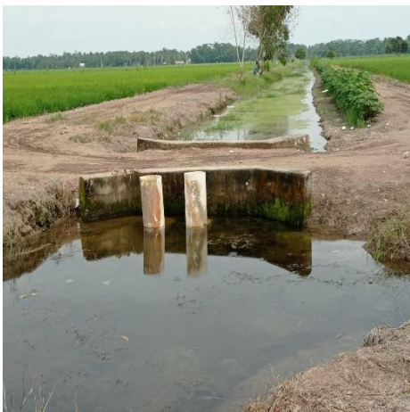
Figures 5 and 6. The completion of the goose-neck sluice
