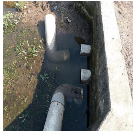
Figures 3 and 4. Gooseneck sluice gates are closed and open in the village Telang Jaya District. Muara Telang Kab. Banyuasin
