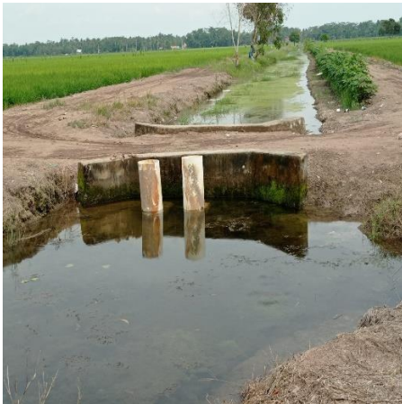
Figures 3 and 4. Gooseneck sluice gates are closed and open in the village Telang Jaya District. Muara Telang Kab. Banyuasin
