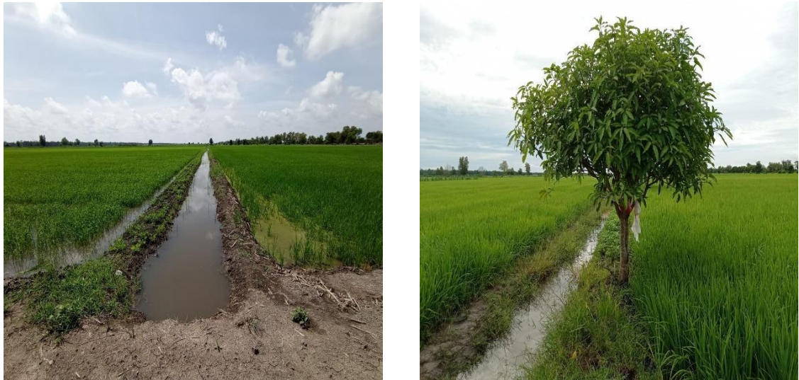
Figure 4.9. Picture of Quaternary Channel in Telang Jaya Village, Muara Telang District Banyuasin Regency
