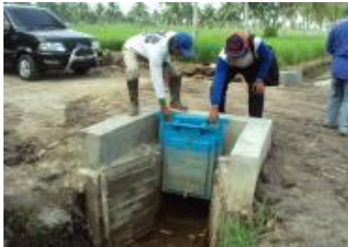
A. Tertiary gate
