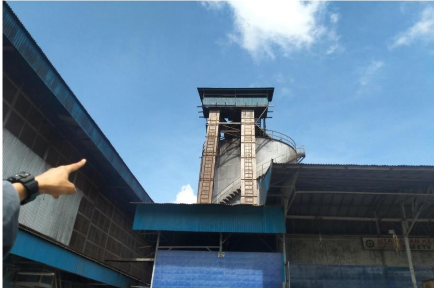
Figure 4.6. Raw Materials Are Brought To The Silo Using Elevator
