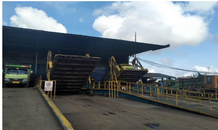
Figure 4.5. Second Unloading Using Hydraulics
