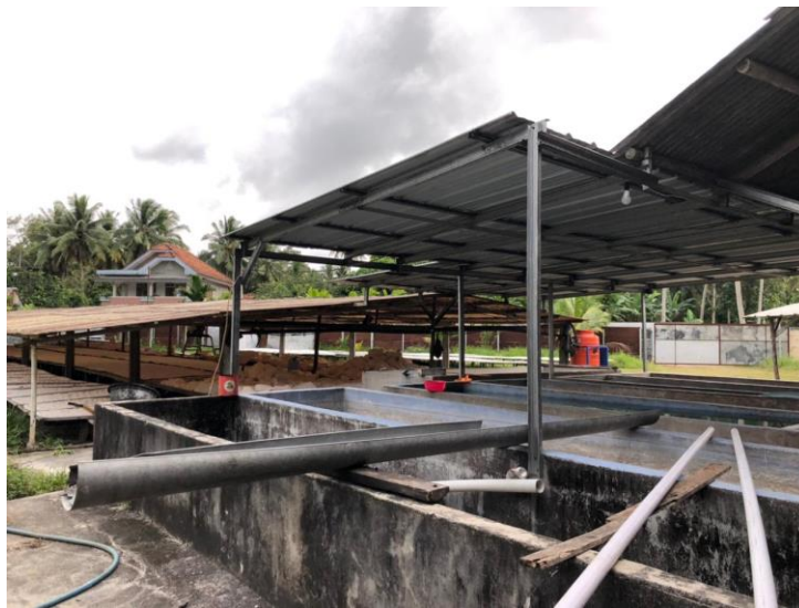
Figure 4.28. View of the Building on the Processing of Sago Palm
