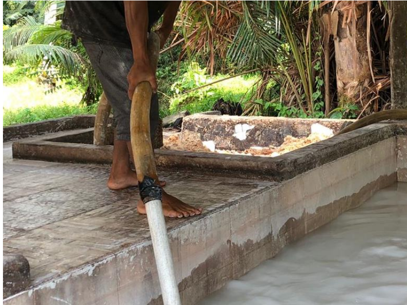
Figure 4.21. Connecting Hose between Pipe and Robin Drive Machine
