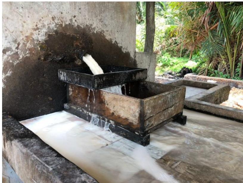
Figure 4.31. Sago Starch Extract Flowing to the Storage Tank
